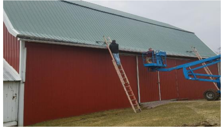
New gutters put on the barn in March!
